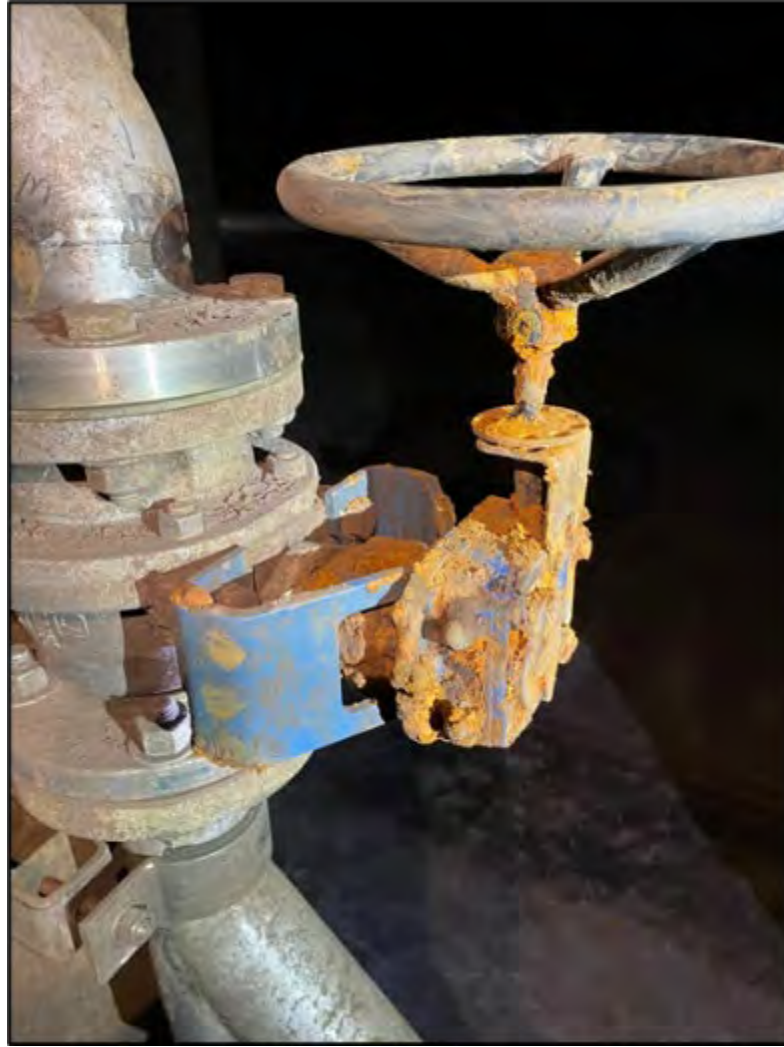
Stainless Steel Valve – Located Inside an Untreated Water Tank
