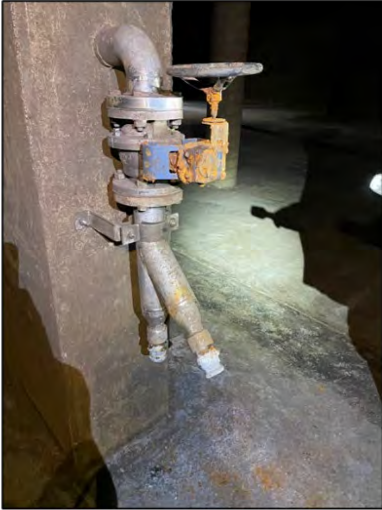
Stainless Steel Valve – Located Inside an Untreated Water Tank
