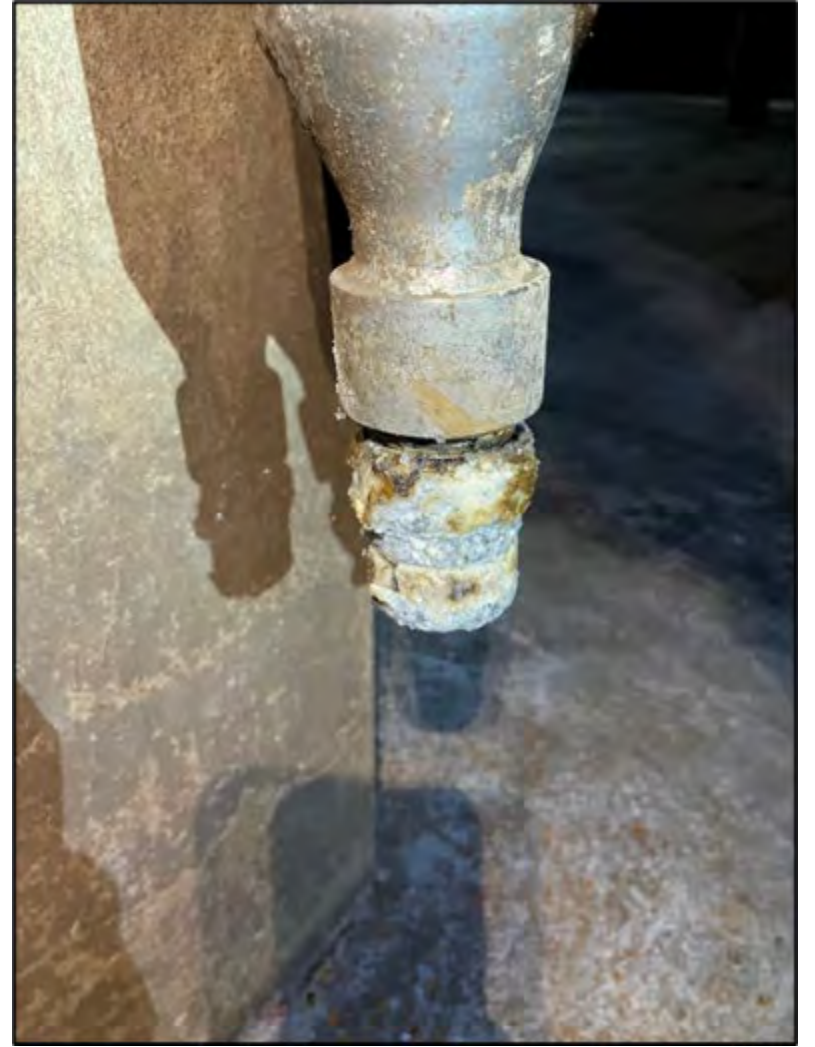
Stainless Steel Valve – Located Inside an Untreated Water Tank
