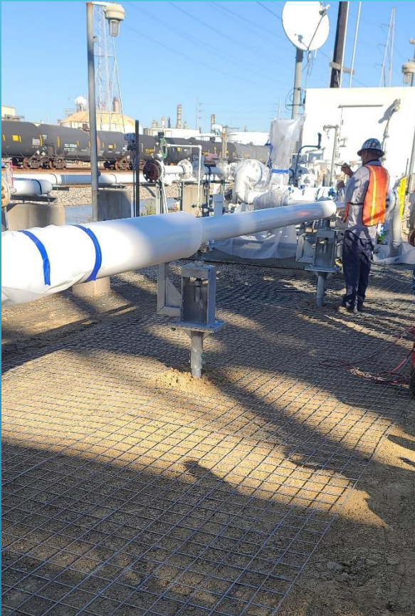
Grounding Mat Work
